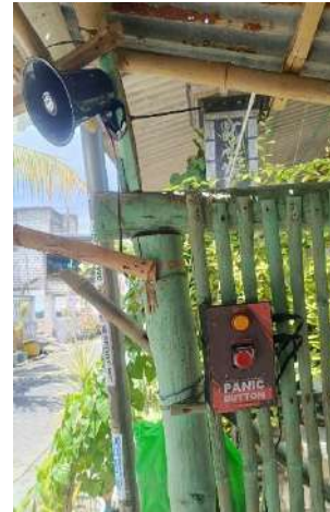
Gambar 14. Instalasi Panel Box Panic Button Di Pos Kamling
