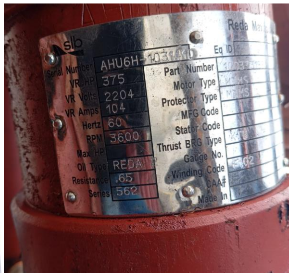
Gambar 1b. Nameplate Motor ESP Sumur 5C-58N (Schlumberger/REDA, Series 562)
