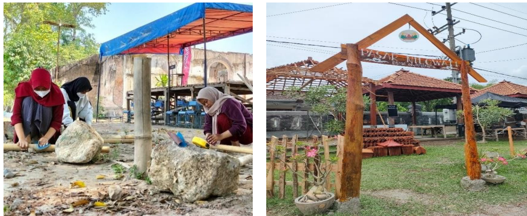
Fig. 1. The process of constructing the entrance gate at Pasar Nilowati
