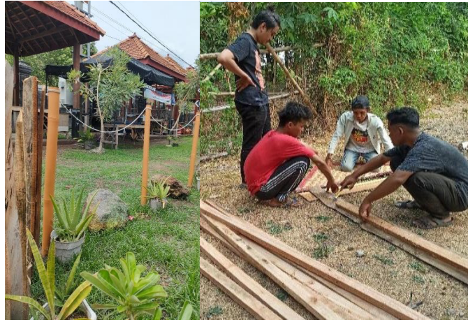
Fig. 2. The installation of bamboo fences for market area arrangement
