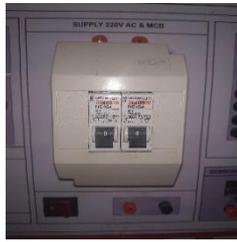
Gambar 7. Gambar MCB (*Miniature Circuit Breaker*)
