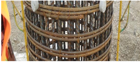
Gambar 7. Beton decking
