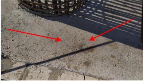
Gambar 8. Garis marking kolom
