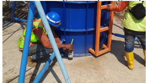
Gambar 12. Proses cek verticality bekisting
