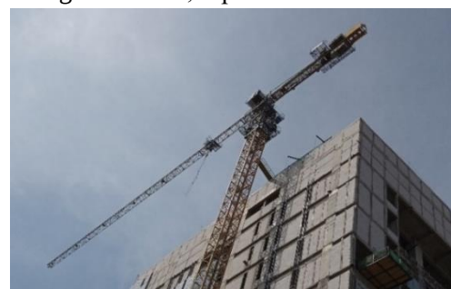
Gambar 5. Tower Crane MCT 205
