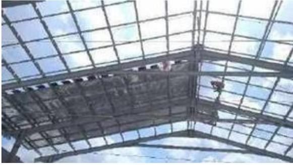
Gambar 26 Roofmesh dan Double Side Aluminium Foil
